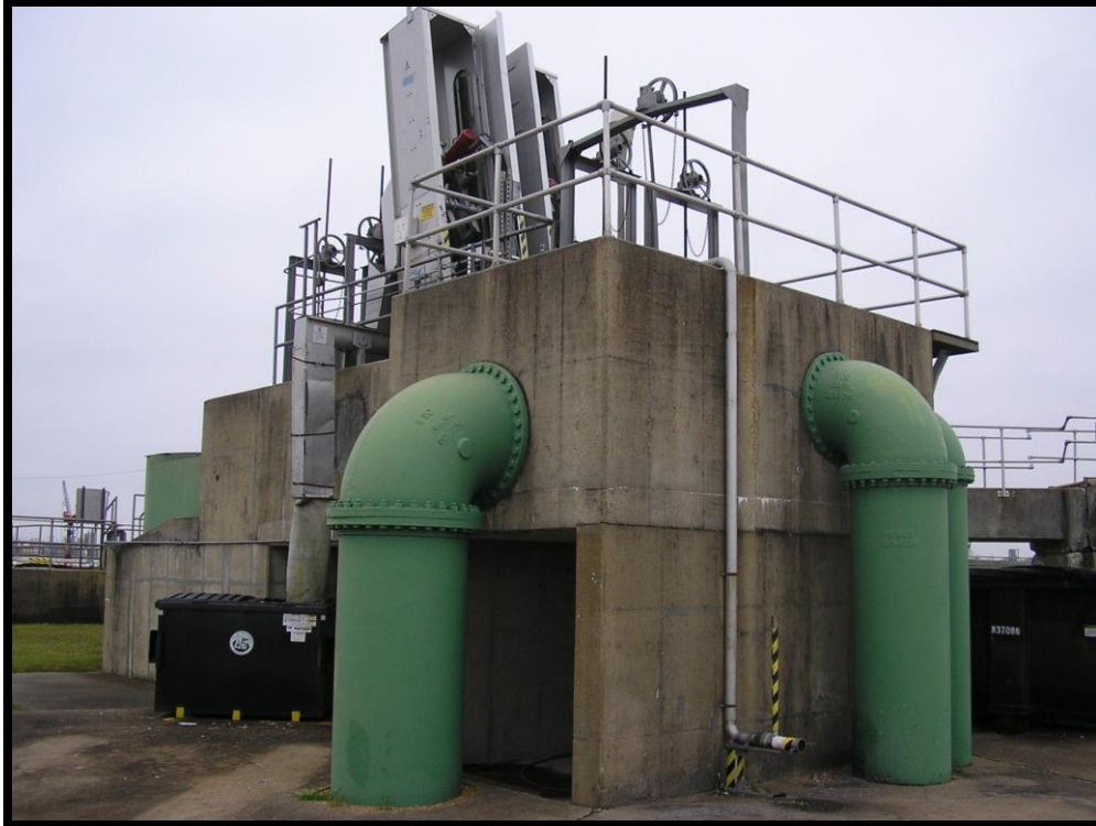
Existing Headwork Structure Showing 36" to EQ Basin, 30" and 20" Influent Force Main
