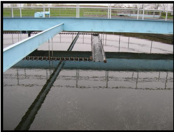
View of Effluent Weir of Original Peripheral Fed Clarifier
