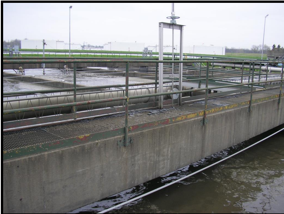
Existing Influent Flow Distribution Channel atop Aeration Basins
